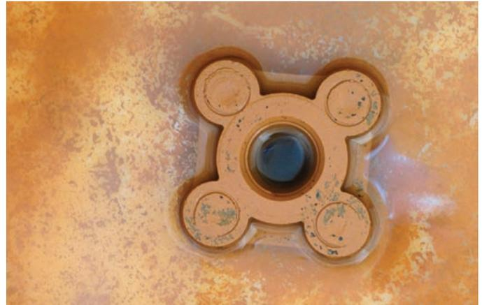
Typically, a tank's drainage opening is slightly above the bottom of the sump. The size of the sump and the area below the drain opening will determine how much residue may remain on the bottom of a tank.
