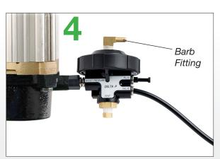
Connect tubing between barb fitting on Delta P and water source upstream of booster pump. Water source is commonly found at the last sprinkler.
